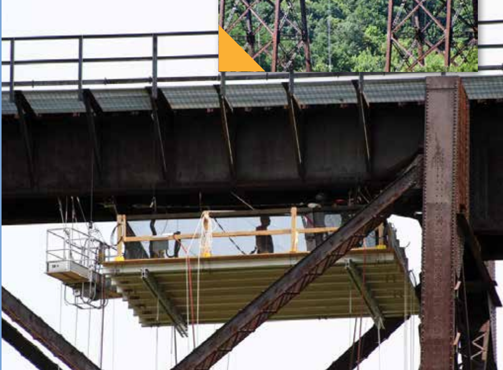
Metro North Railroad Moodna Viaduct Saulsbury Mills, NY Project Scope: Large area float access for structural repair of iron railroad viaduct
