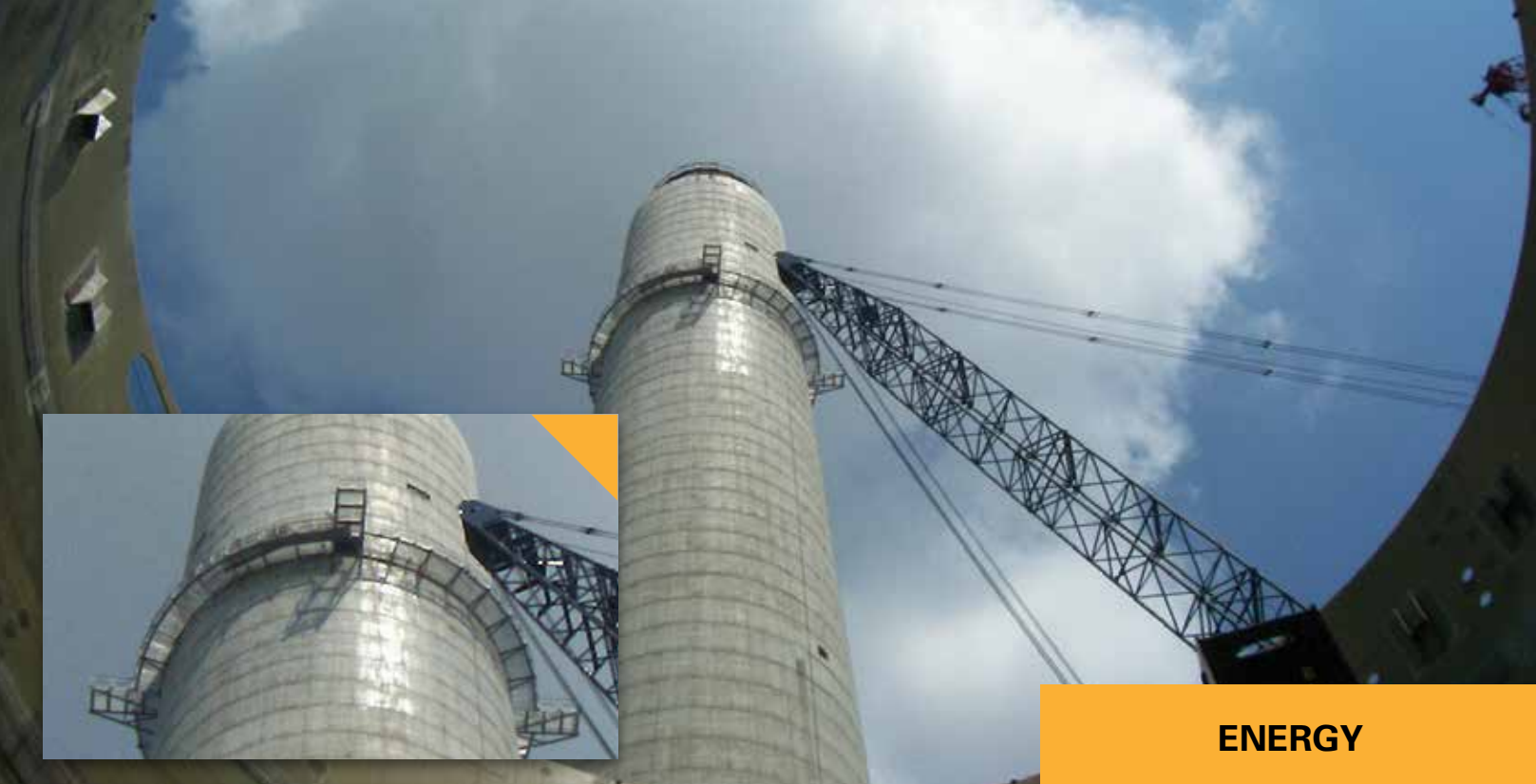
Gulf Power/Crist Plant Pensacola, FL Project Scope: Provide access to the jet bubble reactor's upper tank wall and beams for sanding, joint finishing, and joining beams to tank wall, and to beams to install piping for the cooling process.
