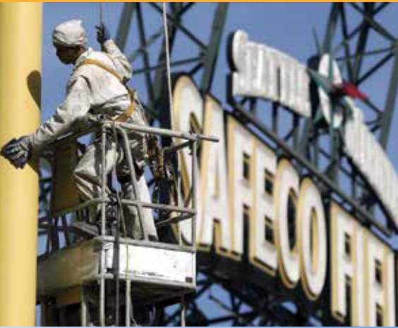
Safeco Stadium Seattle, WA Project Scope: Provided 2 line and single line powered access stages for painting the stadium.
