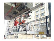
Because this jobsite is located on the windy west bank of the Hudson River, Spider engineered custom catch baskets for electrical cables, double wire rope winders, and dogline modular platforms that eliminated the need for safety lines. These features simultaneously protected workers and the delicate façade from dangling equipment.
