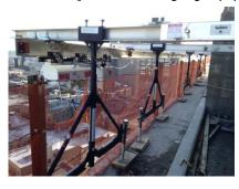
Additionally, Spider's solution included eight SC1500 traction hoists, gantries, max reach assemblies, OBS frames, and a custom trolley for the material hoist controller.
